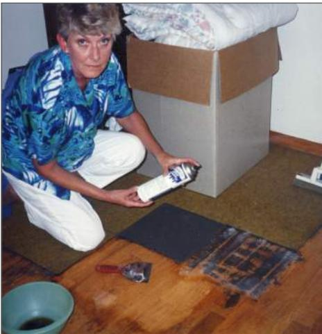
Four square feet in eight minutes; removing the rubber backing, the original varnish & having 100% clean wood that is ready for finishing.
