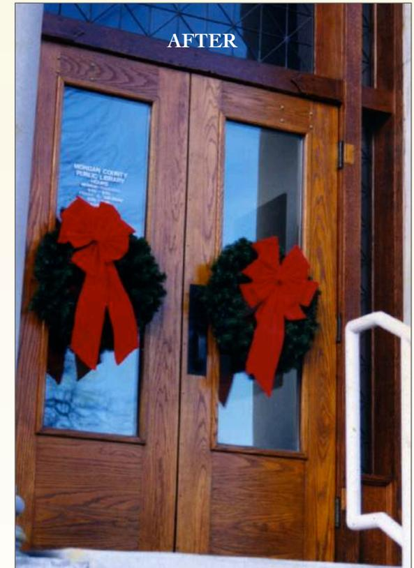
This entire entrance was stripped 100% to bare wood (no damage to patina) using Star 10 'Phase 1 Paste' and Star 10 'Phase 2 Liquid' stripping products. The doors were then refinished with two coats of marine varnish in a total of 15 man hours.
